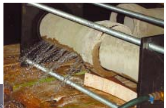
Water tightness test showing that the pipe barrel leaks before the joint.
